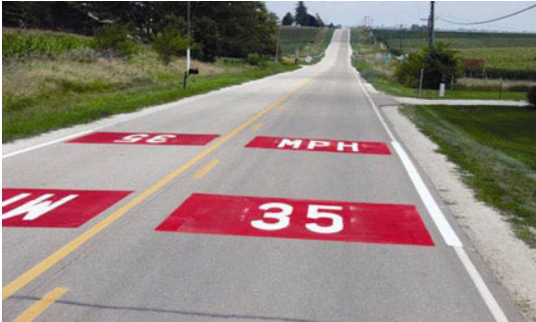
Entrance Treatment Using "35 MPH" Legend with Red Background
