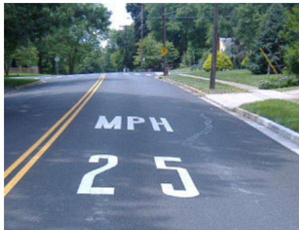
Speed Limit Pavement Legend (MUTCD Section 3B.20)
