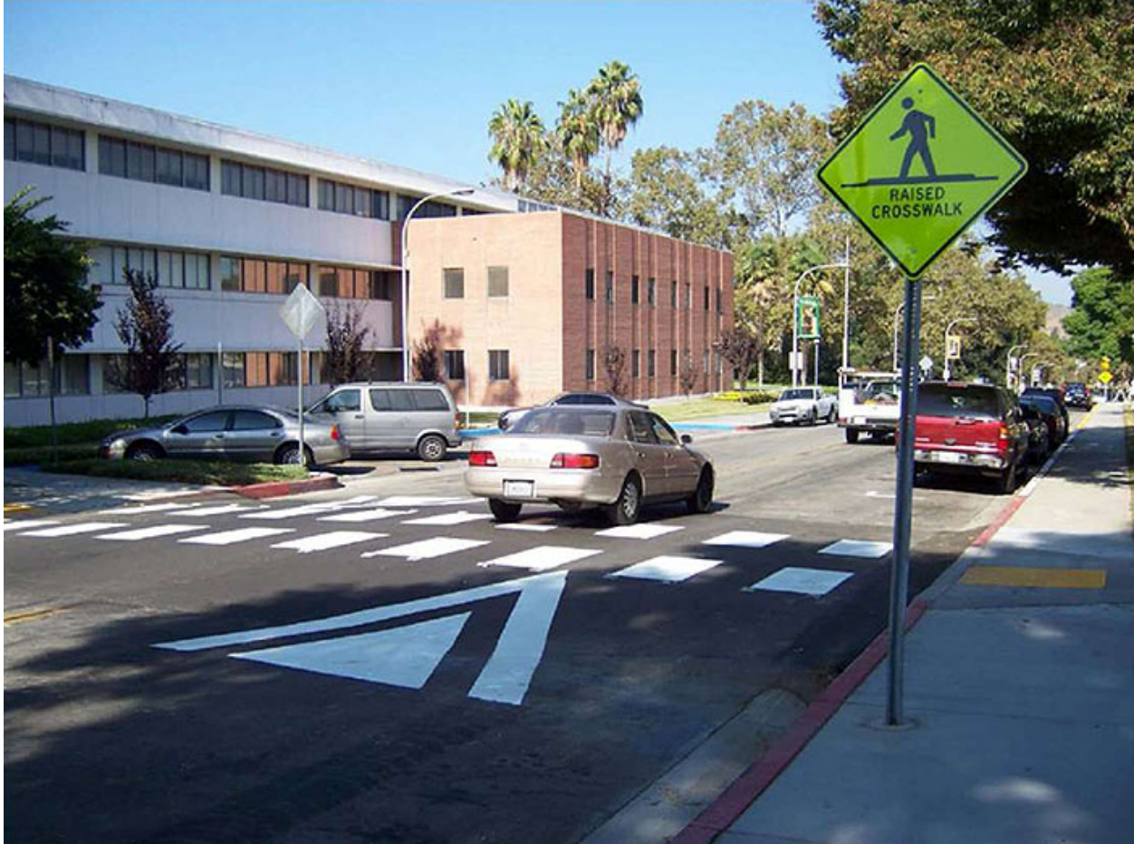
Figure 3.14.2. Typical Raised Crosswalk Application
