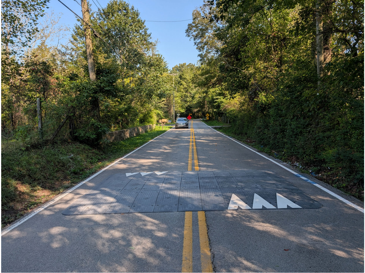
Typical Speed Table Application
